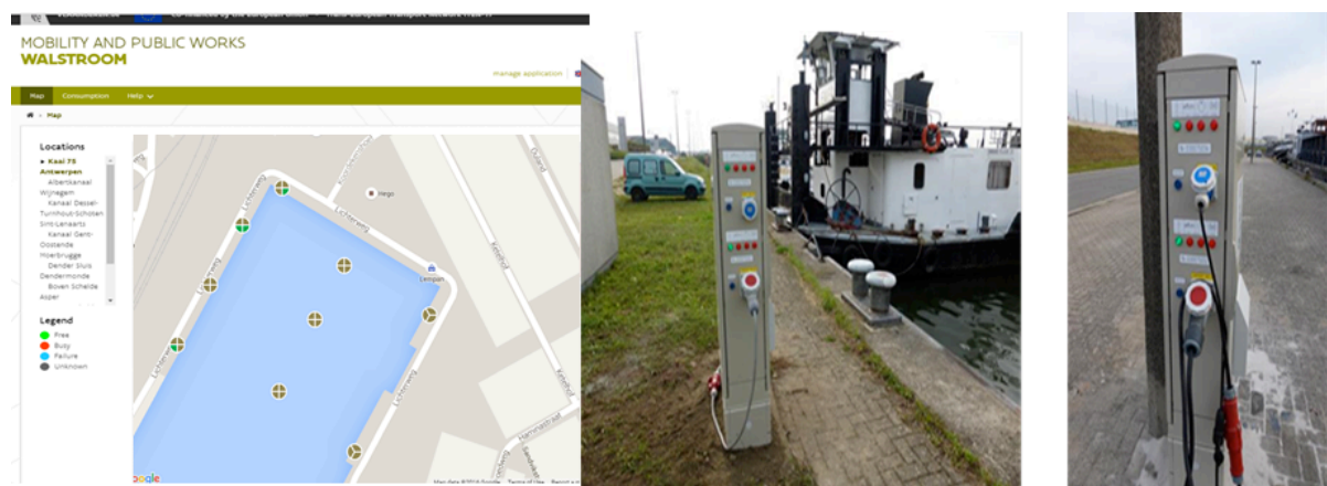
Figure 5.2 Shore power installations (low voltage) at quay 75 in Port of Antwerp
