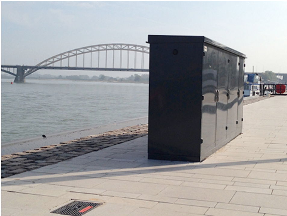
Figure 4.2 Example of an OPS cabinet on Waalkade in Nijmegen
