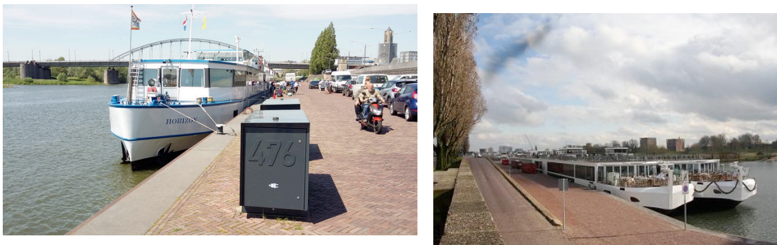
Figure 4.5 Overview of river cruise berth Nieuwe Kade Arnhem with OPS cabinets
