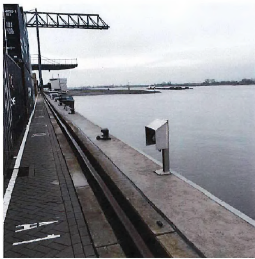
Figure 4.7 OPS sockets on BCTN quay (source: BCTN)
