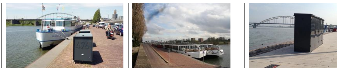
Example of an OPS cabinets in Arnhem and Nijmegen
